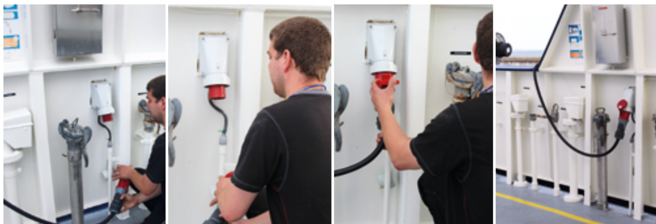
Staff connect to the shore power supply to commence charging the battery bank.
