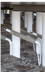
Siphon pilings used to support the pool. Credit: kengrahphotography.com.
