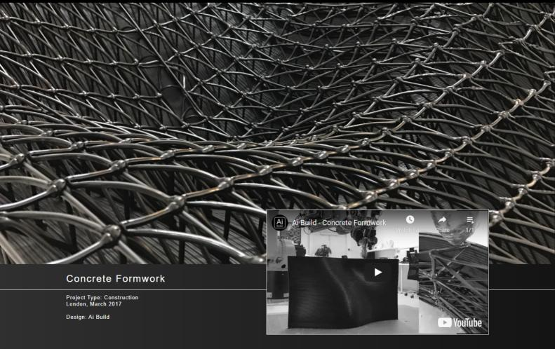
This project investigates AiBuild's ongoing development on 3D printing custom molds. Main advantages for using 3D printed formwork in construction are increased design flexibility and zero material waste. Thanks to its light and robust structure, this technique can reduce labour intensive work.
