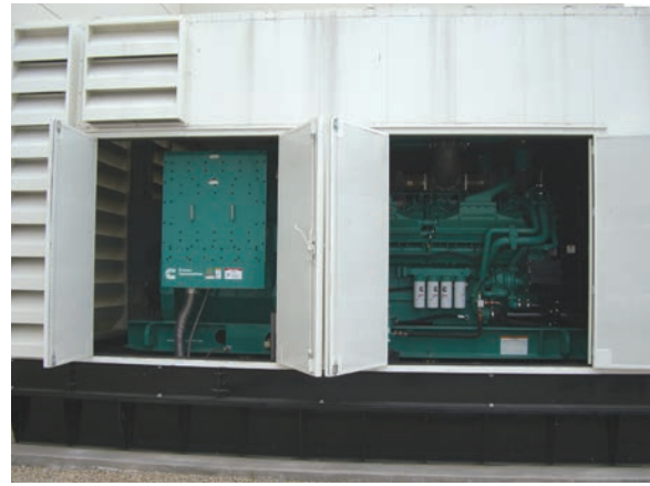
Standby power is provided by two 2 MW DQKAB generator sets in a sound attenuated housing.
