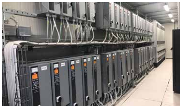
VFDs in the Sarlux SWRO plant
