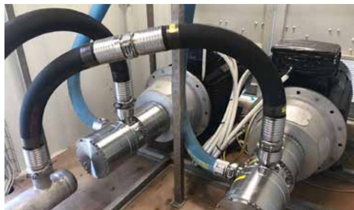
APP 86 pumps in the Sarlux SWRO plant
