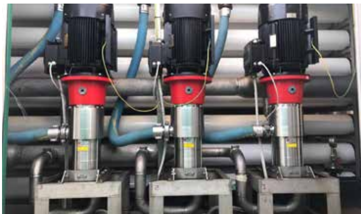
iSave 70 energy recover devices in the Sarlux SWRO plant
