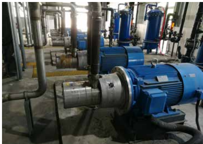
Danfoss APP pumps operating in different trains at Chuan Ning Biologicals ZLD treatment plant
