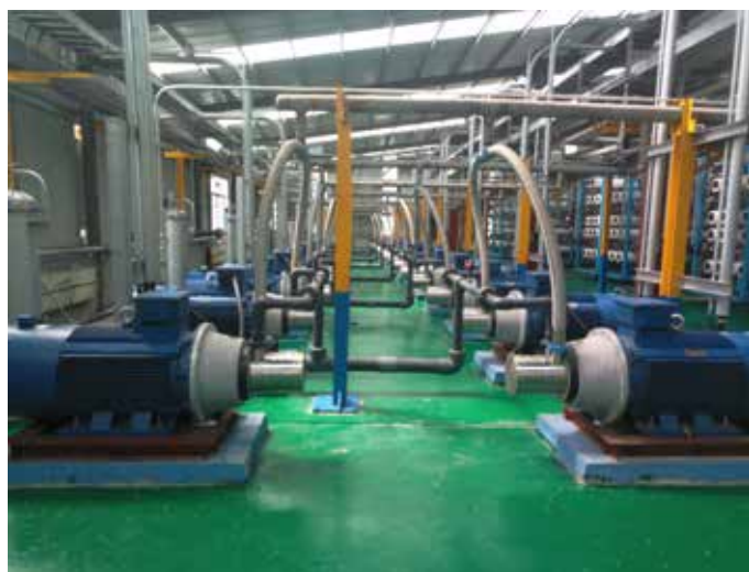
Danfoss APP W 24 pumps operating in parallel
