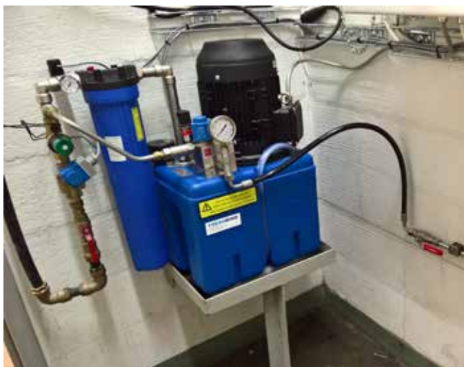
UPW pump unit using a PAH 10 pump
