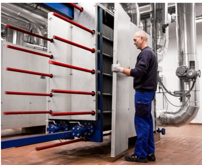
Replacing the old heat exchangers' plates with new ones at AffaldVarme Aarhus
