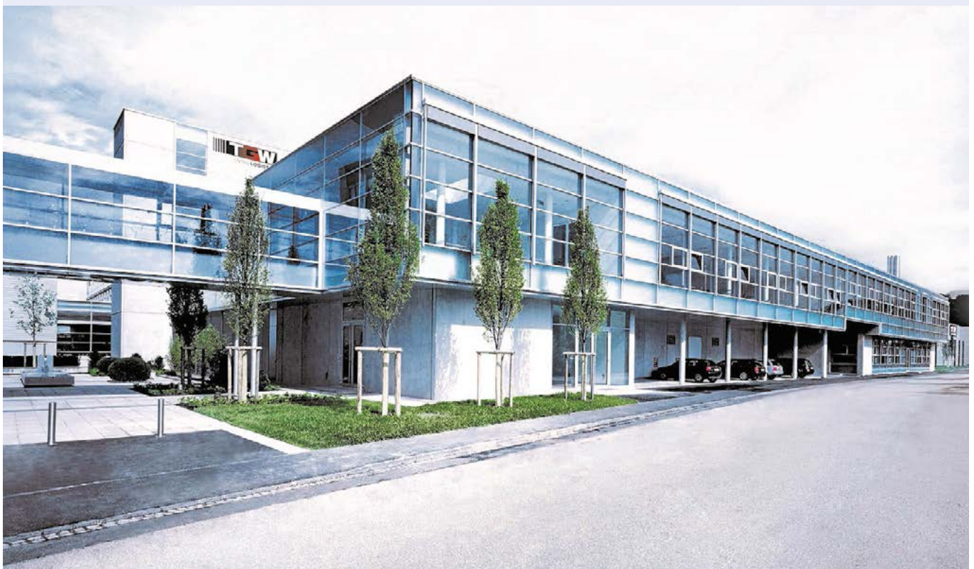
The TGW Logistics Group headquarters in Wels, Austria
