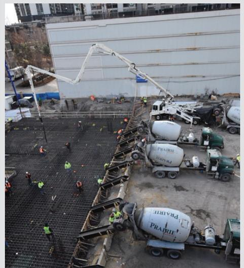
Continuous mass concrete pour over SmartRock™ wireless sensors installed on rebar
