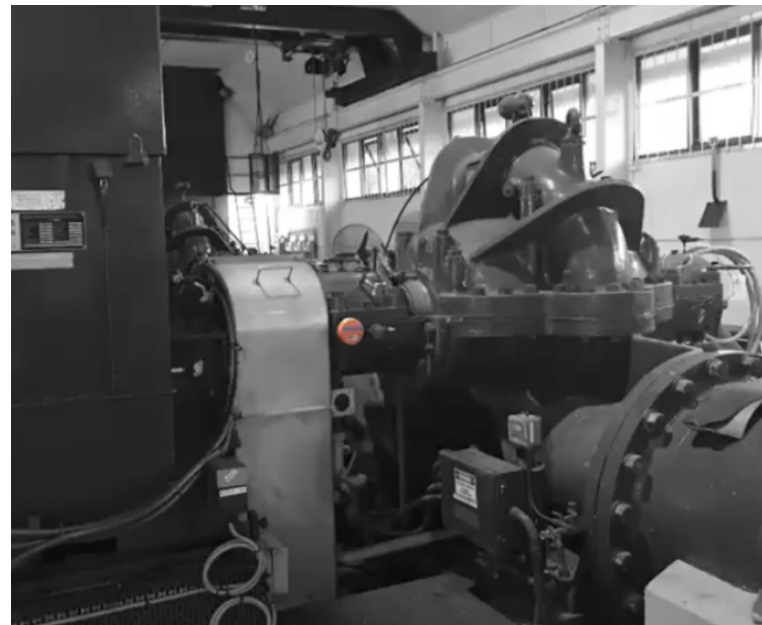
Parsons & Peebles 1800kW Induction motor and a Thompsons horizontal split-case pump with an installed FitMachine.
