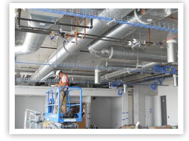
file directly to the Trimble Total Station and Nomad field device. Using a scissor lift and the Trimble field devices, one field person can move from position to position, locating pendant points directly on the structural elements then shoots the anchors in, thus eliminating the need to lay points out on the floor and transpose them back up to the ceiling. In addition, the new process only takes about two hours to set up and export to TPC.
