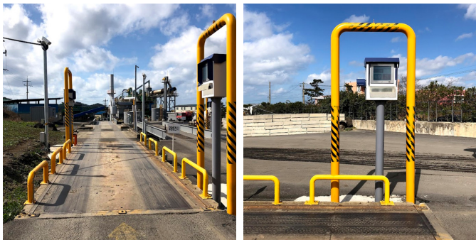
Weighbridge and automatic measuring equipment installed at the entrance of a waste disposal facility
